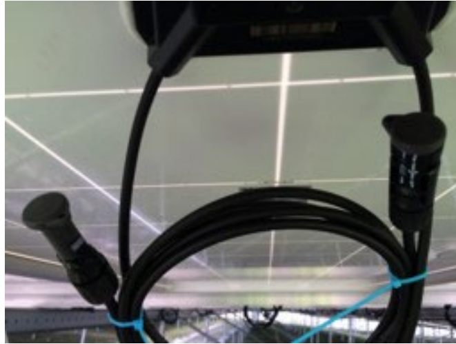
Example of a PV modules with un-matted connectors with protective caps (Picture/Illustration of Stäubli, Switzerland)
